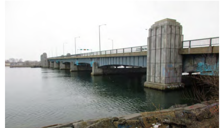
View towards General Edwards Bridge
