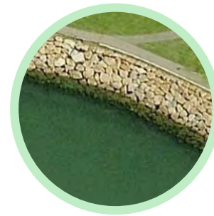
REVETMENT WALL stone block
