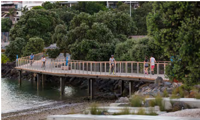
Potential for raised boardwalk over eroded edge
