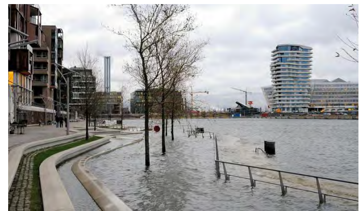
Waterfront areas designed to be flooded and returned to use
