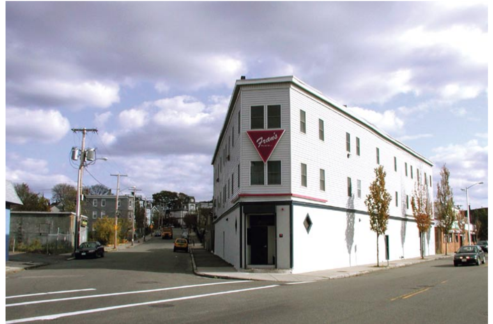
WASHINGTON STREET AT SAGAMORE STREET - BEFORE
