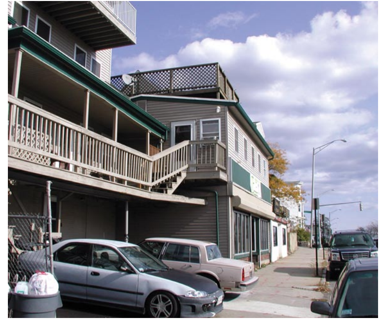
THE LYNNWAY NEAR NEWHALL STREET - BEFORE
